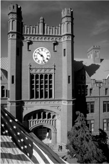
Administration Building, University of Idaho Photo Courtesy: University of Idaho
