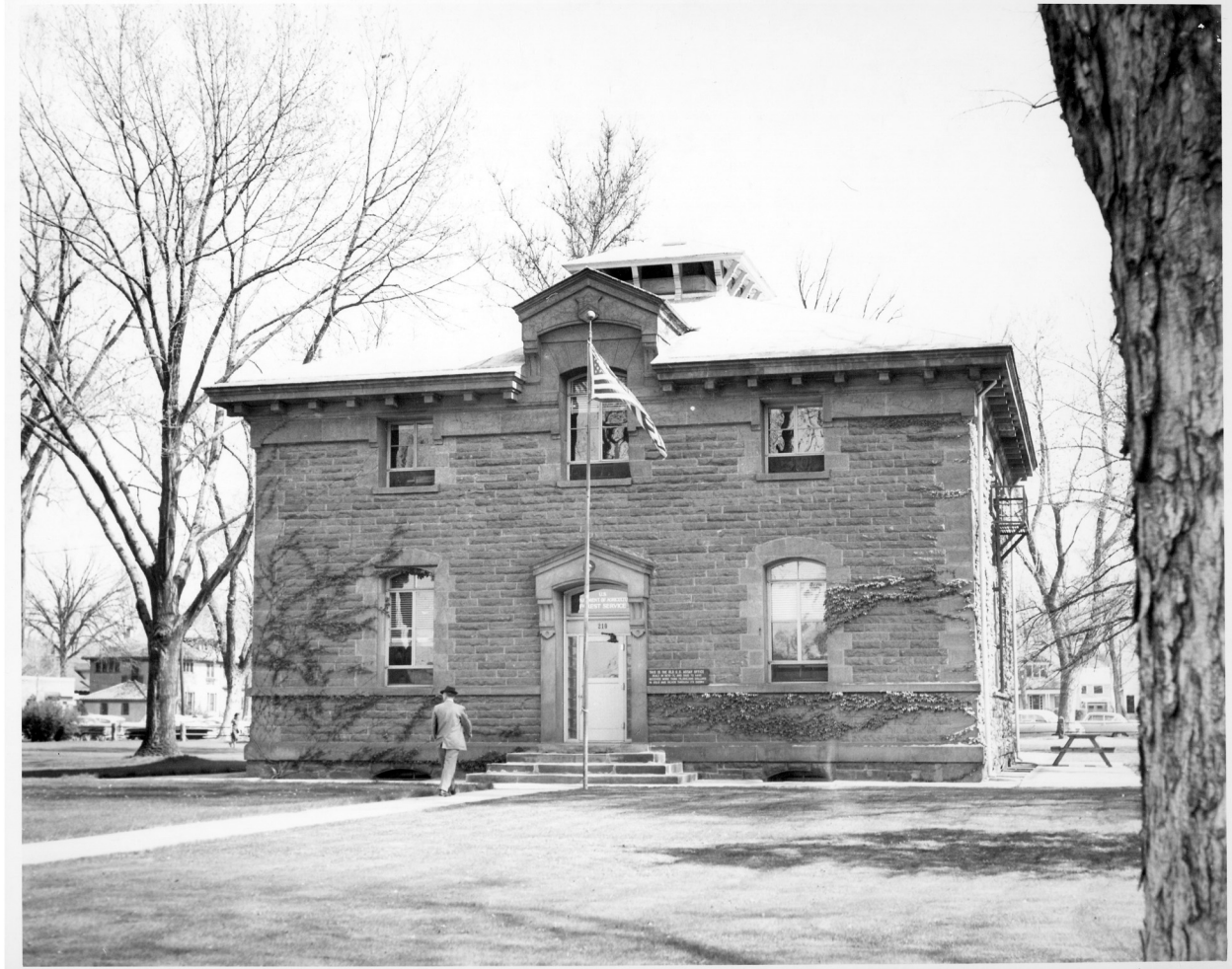
61-79.2 U.S. Assay Office. Later U.S. Forest Service headquarters. Built 1870-1871. Photo by H.S. Swinney, April, 1961.jpg
